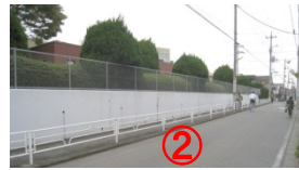
② 白壁と金網 White wall & wire mesh fence
